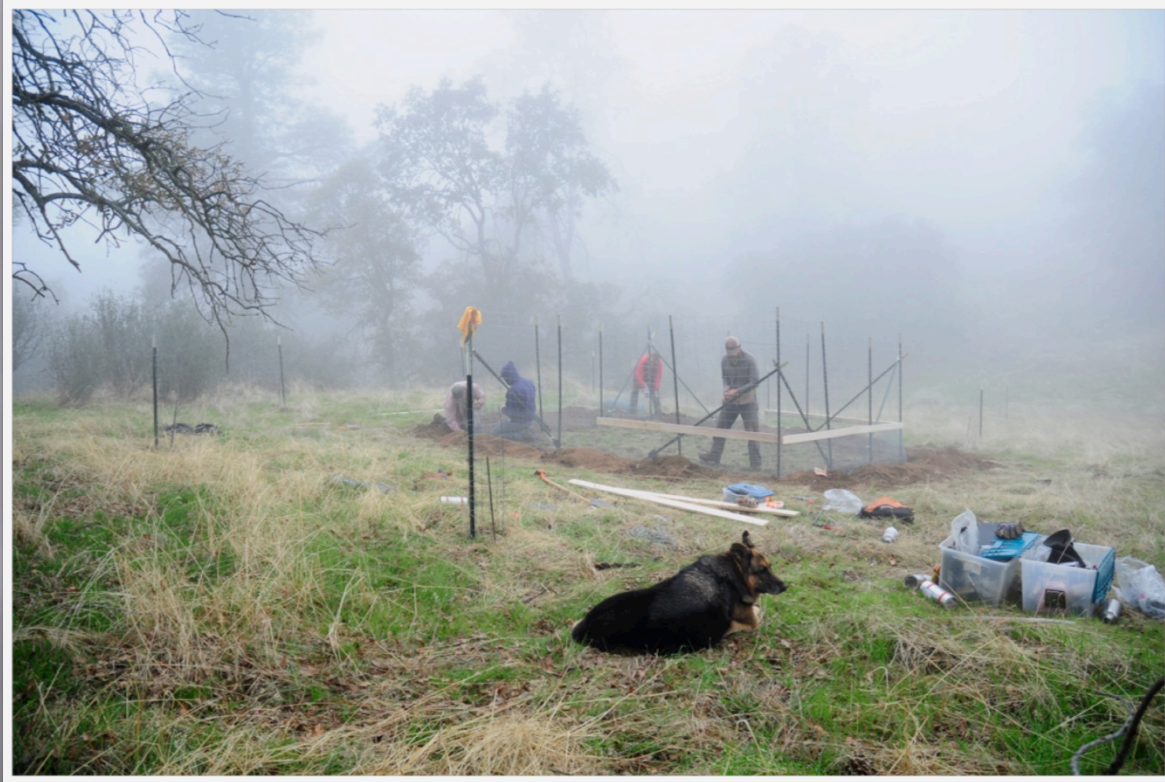
Fencing and Rodent-proofing
