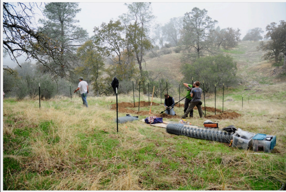
Trenching and Pounding
